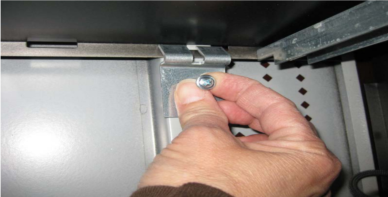
Screw into place using self tapping screws included.
